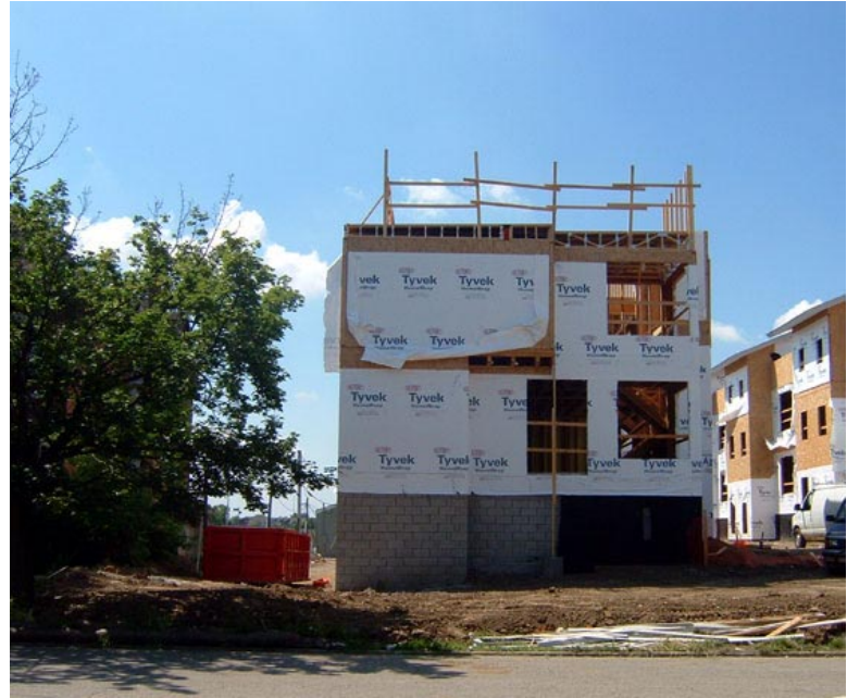
Framing as of 6/20/06
