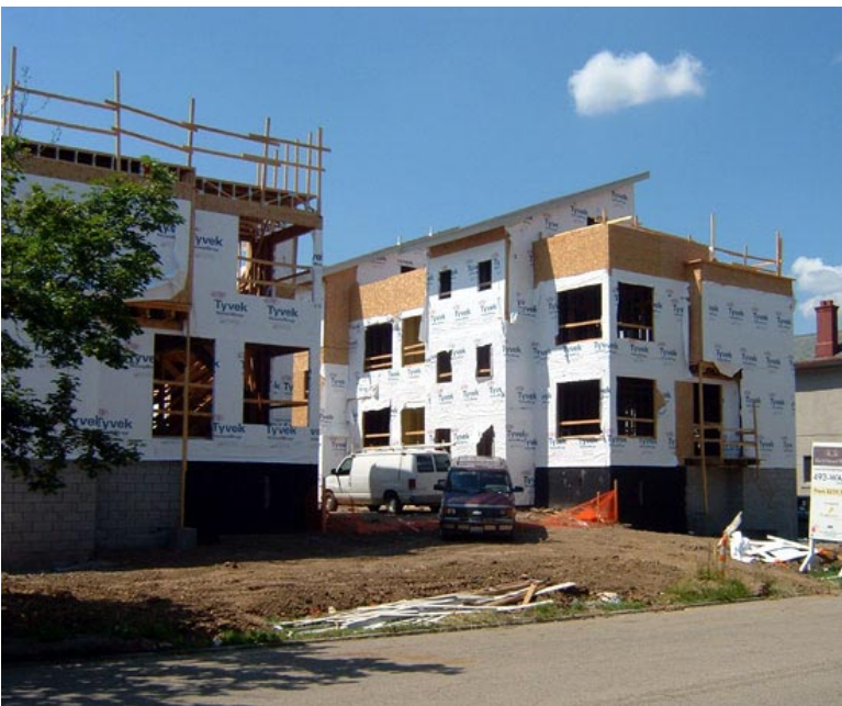
View from Rich Street
