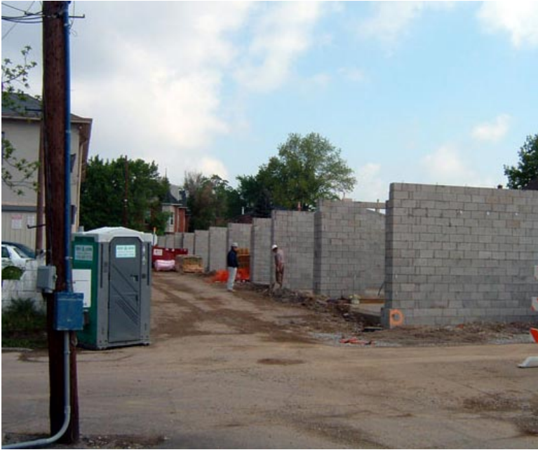
Block Work Complete
