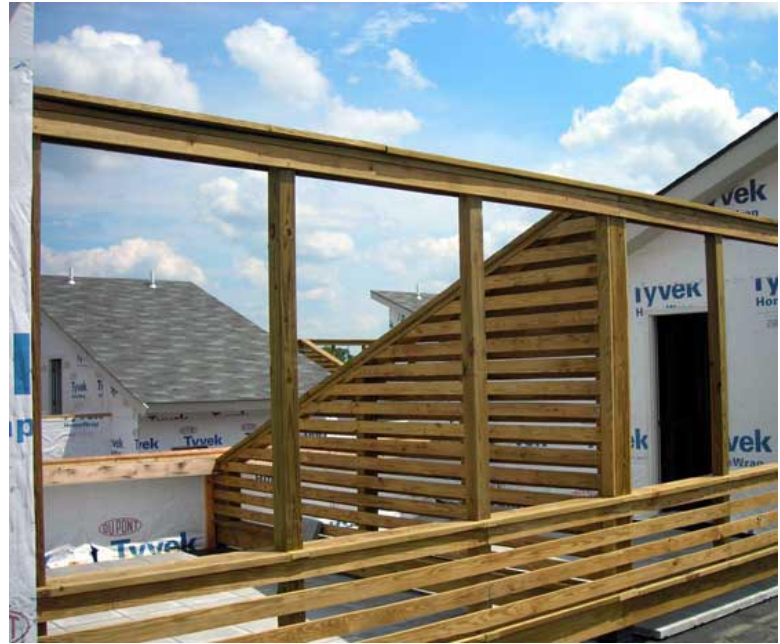
Roof Top Deck
